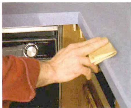
A light sanding completes the job. The edge of the molding should be flush, or a bit high. If high, sand flush with 220-grit paper. Don't sand into the back of the laminate.
